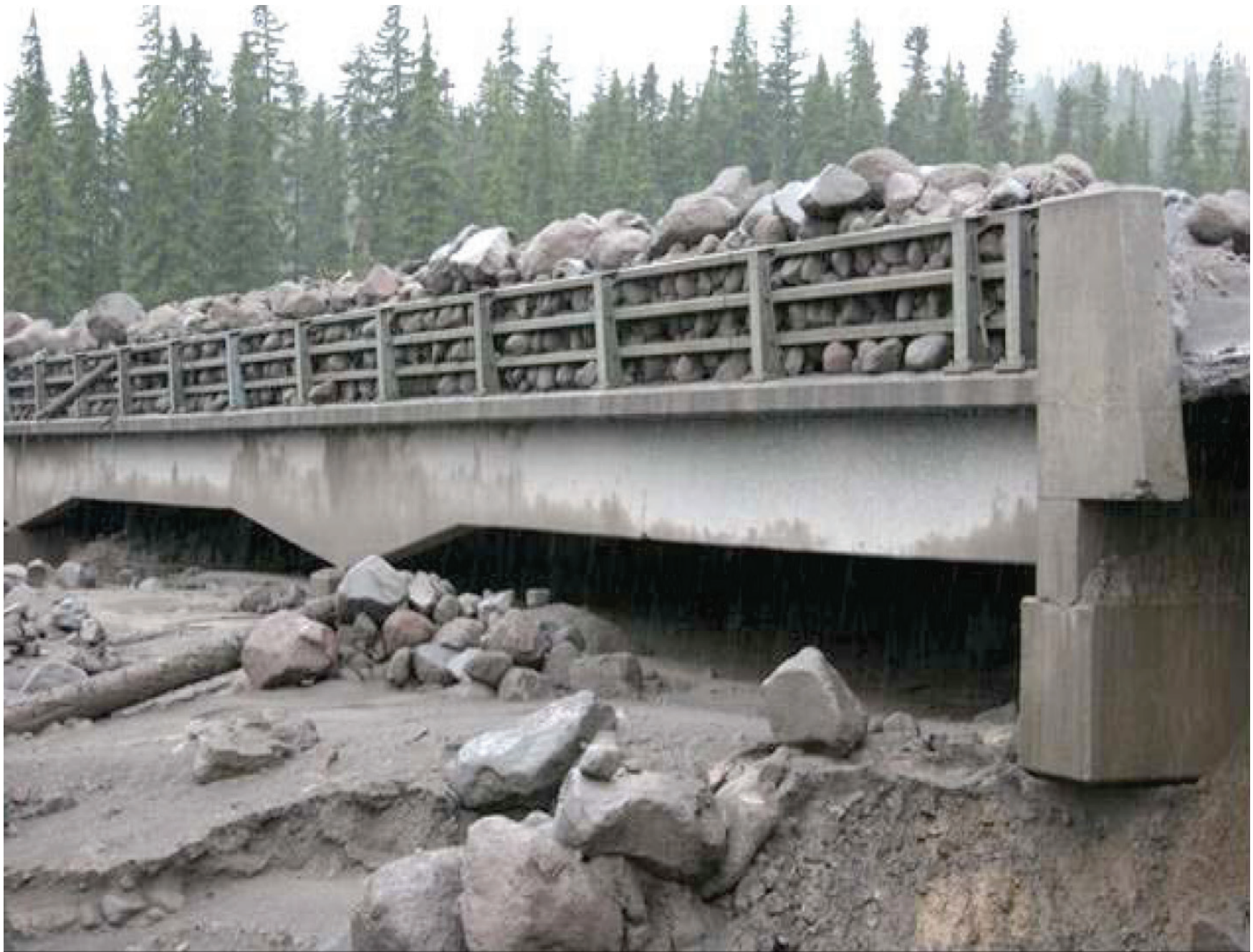
3. Hwy 35 bridge over White River completely plugged underneath by 25 ft of rock, and the bridge itself buried. This is the downstream side.
