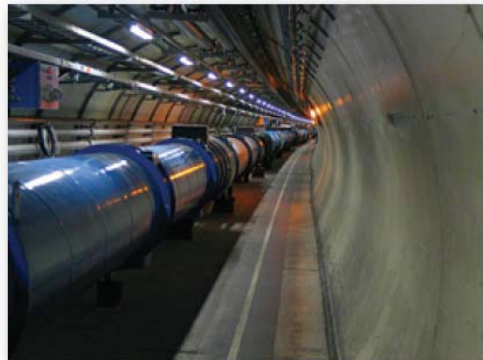
Accelerator Magnets in the LHC Tunnel
